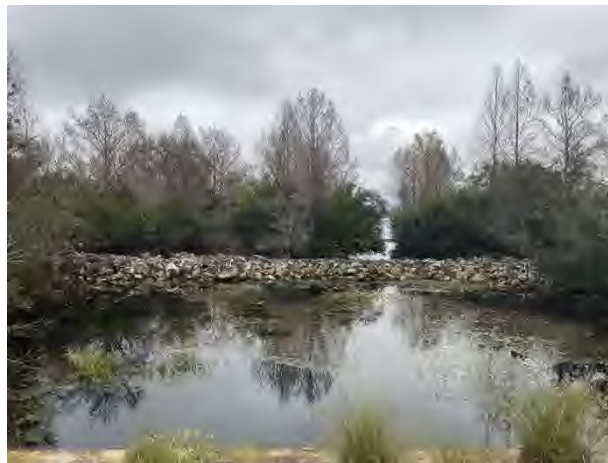
Rip rap and concrete weir
