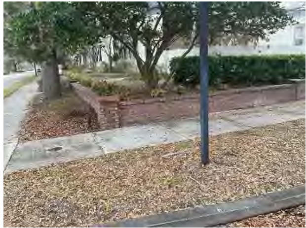
Masonry retaining wall
