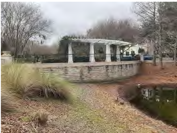
Masonry retaining wall
