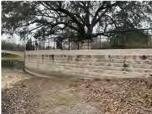
Masonry retaining wall
