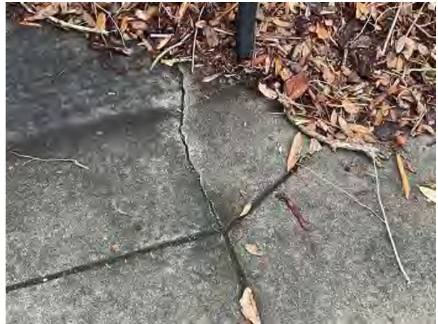
Sidewalk cracks
