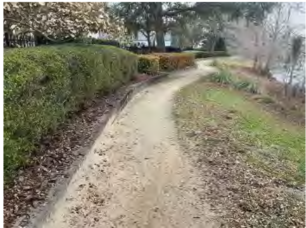
Masonry retaining wall
