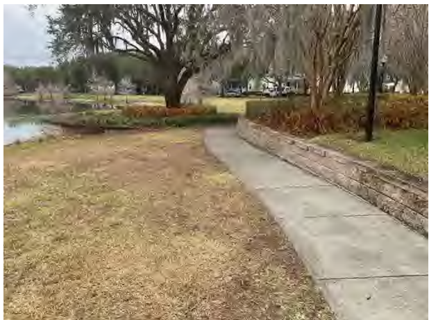
Masonry retaining wall
