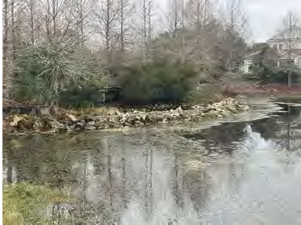
Rip rap and concrete weir
