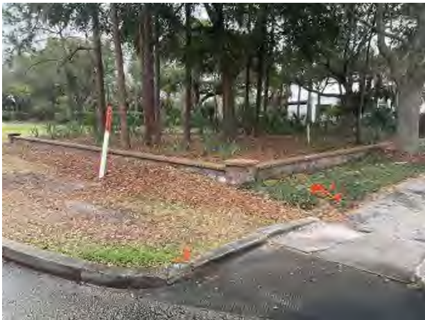
Masonry retaining wall
