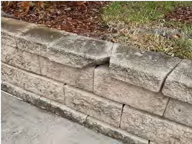
Masonry spall
