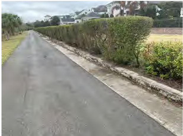
Masonry retaining wall
