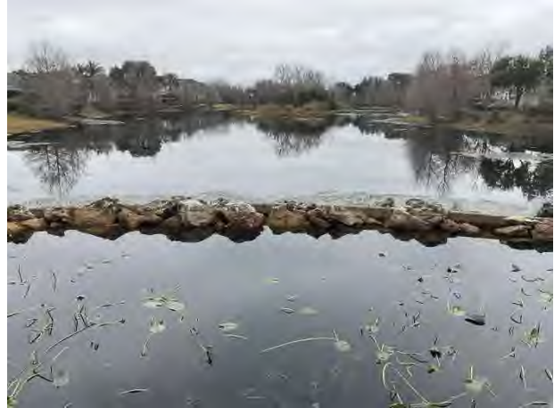
Rip rap and concrete weir
