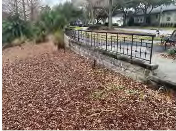
Masonry retaining wall
