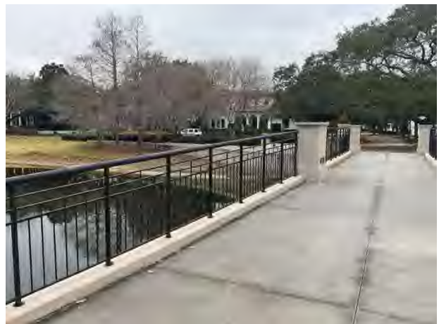
Railings over you at bridge
