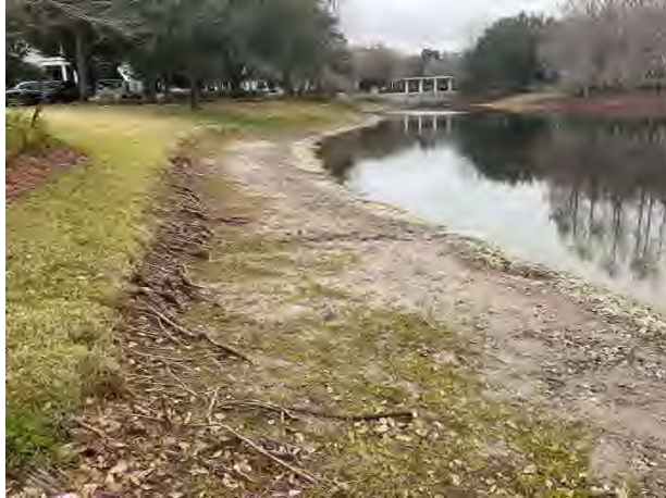
Minor shoreline erosion
