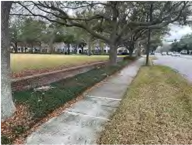
Masonry retaining wall
