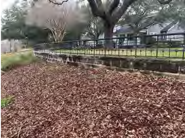
Masonry retaining wall
