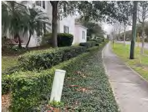
Perimeter wall overview
