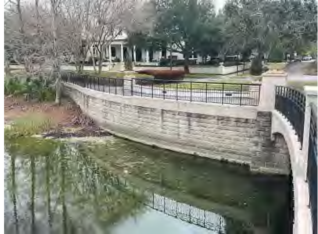
Masonry retaining wall
