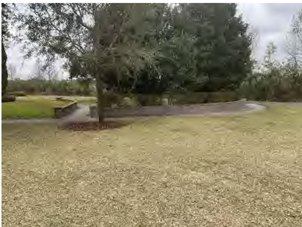
Masonry retaining wall
