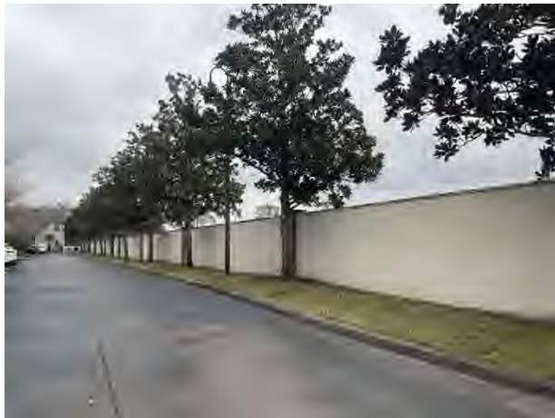
Concrete perimeter wall overview
