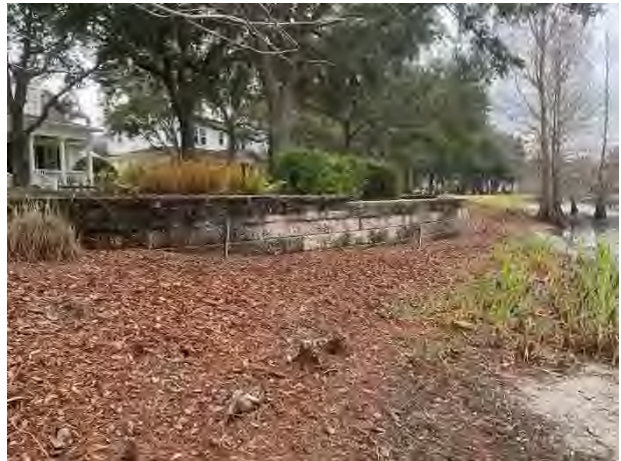
Masonry retaining wall
