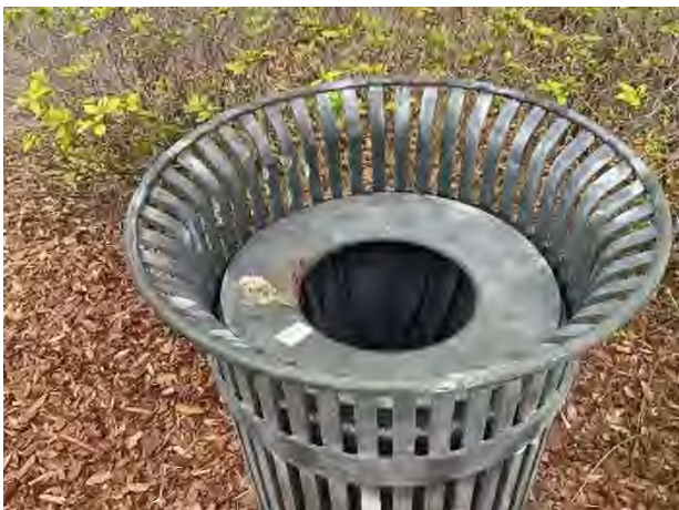
Rust and finish deterioration
