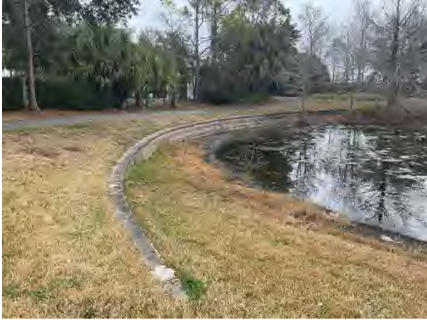
Masonry retaining wall
